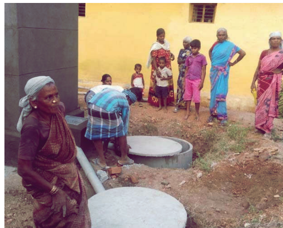
SCOPE built sanitation units that use the tiger worm technology of decomposing waste.
